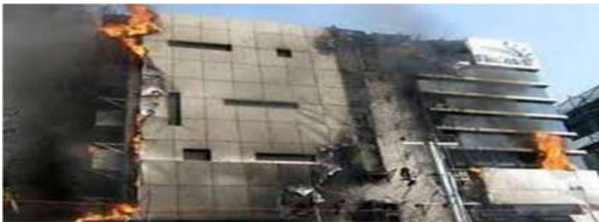
Figure shows fire accident
