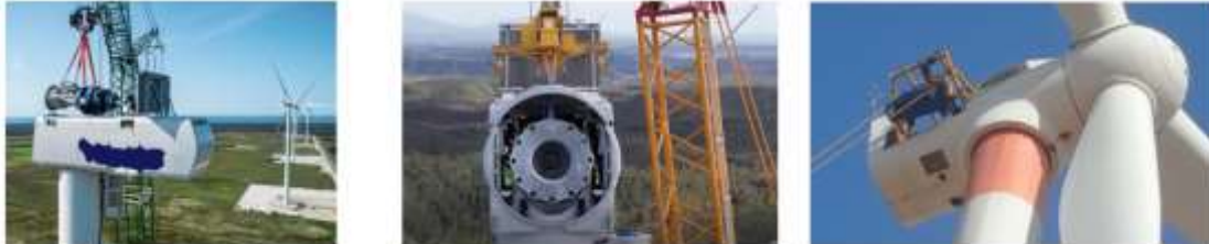
Fig. 4 Work at height activities drive train installation, hub installation, generator replacement.
