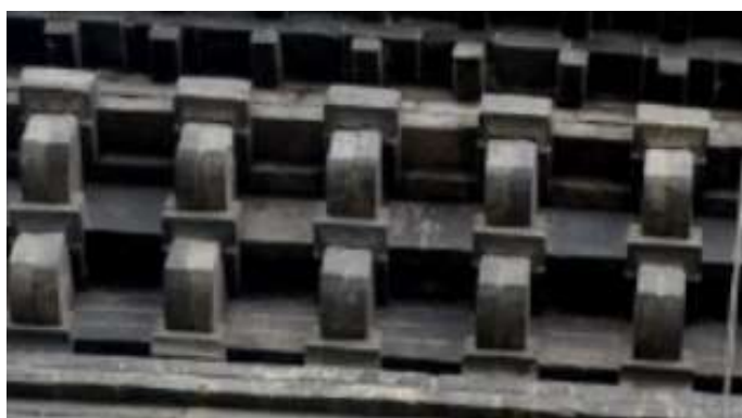
Fig. 26 Parallel transversal arms, Northern Song - Fusheng Temple Pagoda, Shangqiu, Henan
