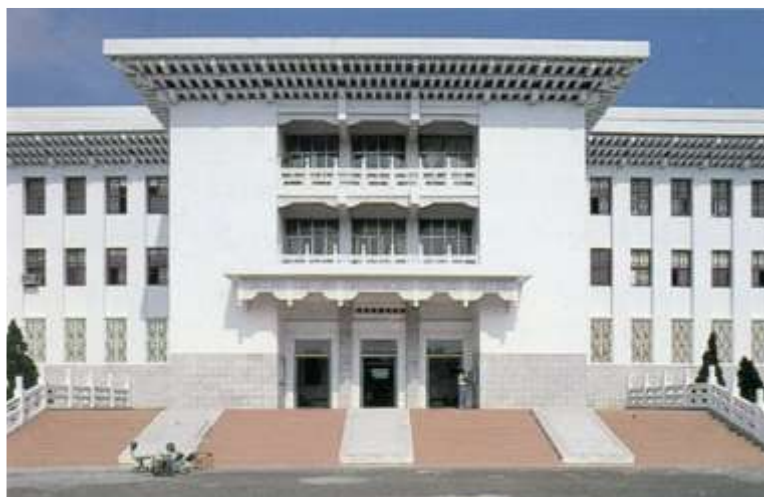
Figure 14 Tamkang University Science Building, Taiwan
