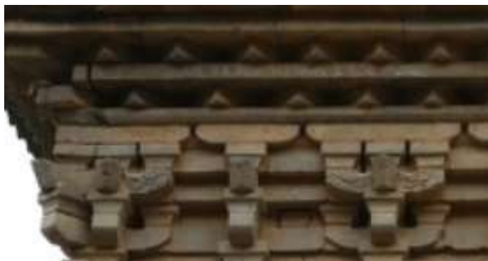
Fig. 27 Individual brackets, Northern Song Dynasty - Jingde Pagoda, Hu County, Shaanxi
