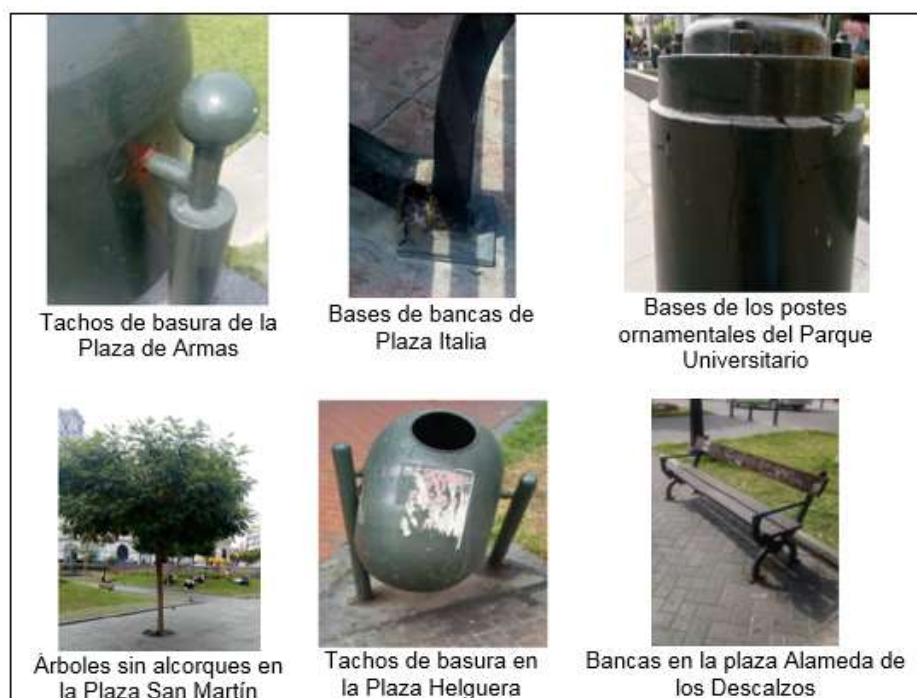
Figure 1. Main failures in urban material in squares and parks in the Historic Center of Lima, 2019.
