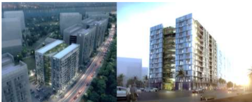
Fig. 3. Residential Buildings (Jawaher Dijla Residential) [10].
