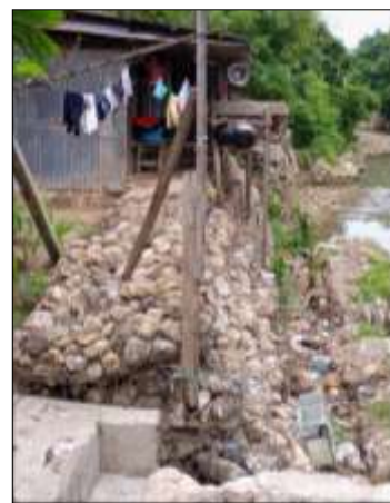
A community's retaining wall (Airmata, Mantasi)
