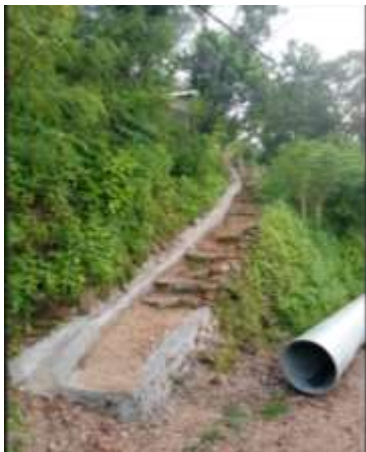
A shortcut way to other region when flooding (Mantasi)
